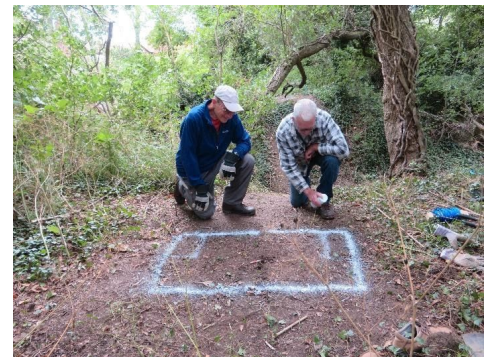
Stan and Brian marking out the foundations for the bridge footings
