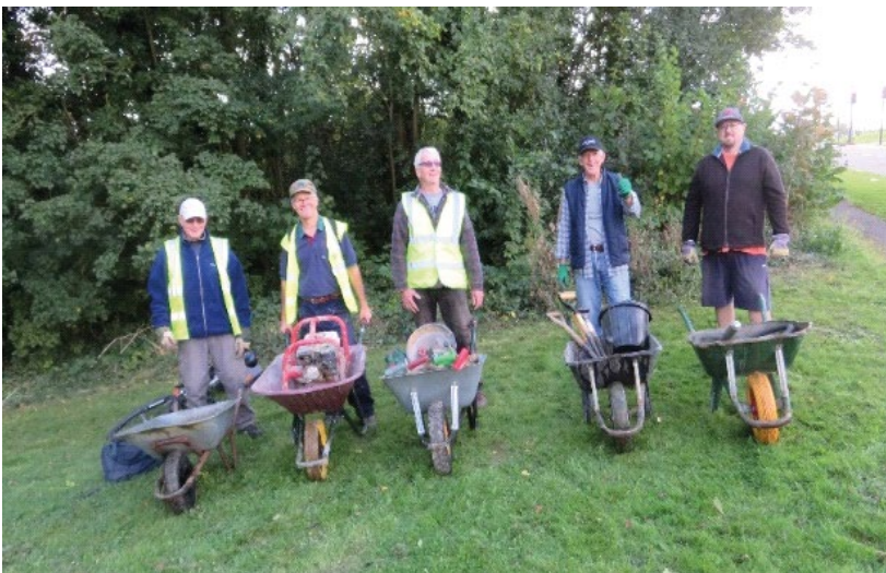
The 'barrow gang', led by Brian Lindsay (centre) that transported the readymix concrete.
